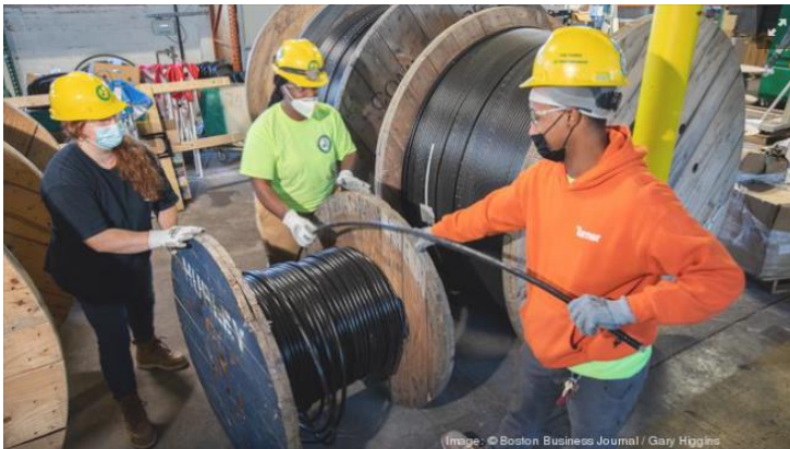
Sullivan & McLaughlin employees Jessica O'Donnell, Kanitra Porch and Jerrell Adams re graduates of Building Pathways Pre Apprenticeship Program and are current members of IBEW Local 103.
