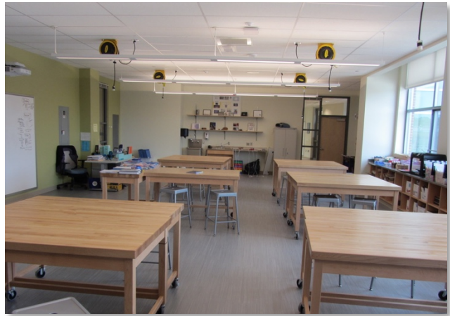
Ceiling bar (left) and electrical drops (right).
