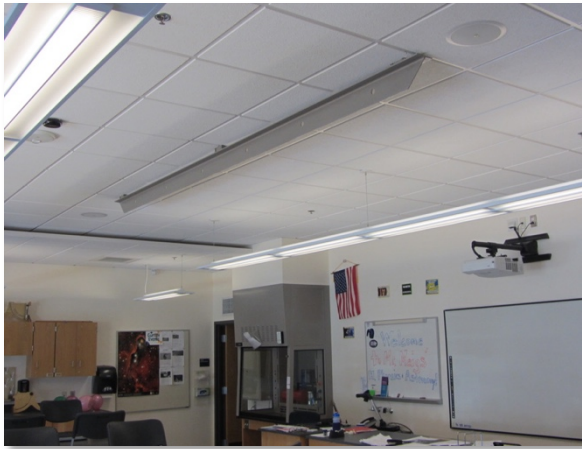
Ceiling bar (left) and electrical drops (right).
