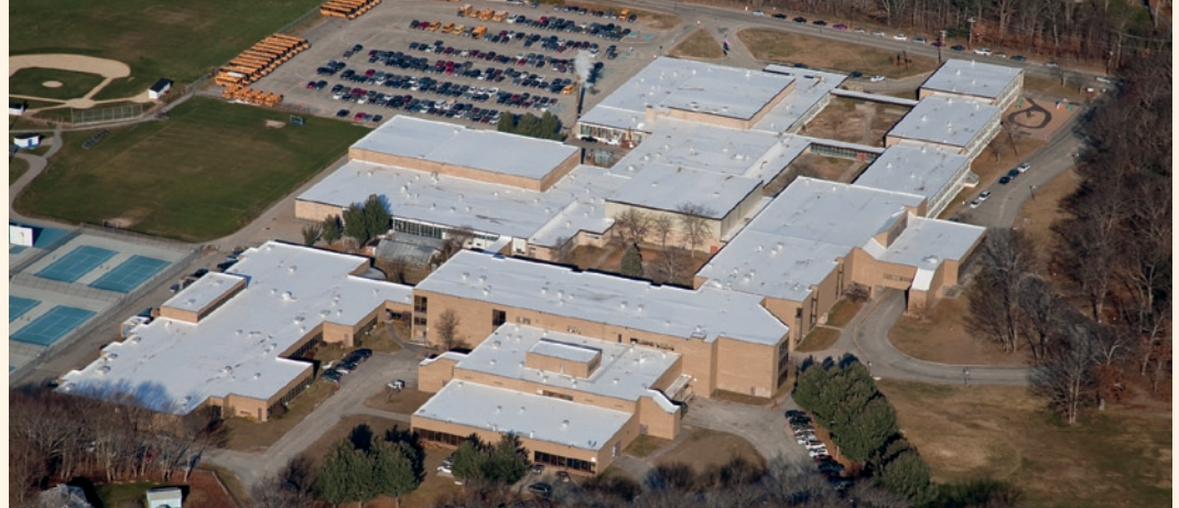
Attleboro High School Roof Repair
