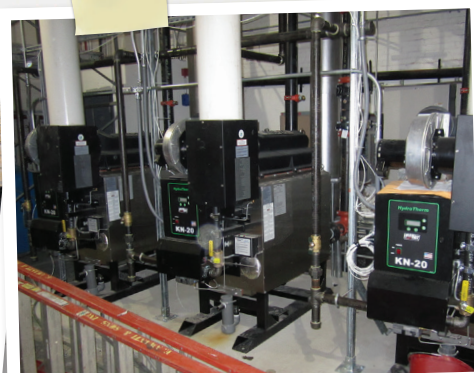
NEW BOILERS WERE INSTALLED AT SALEM'S SALTONSTALL ELEMENTARY SCHOOL
