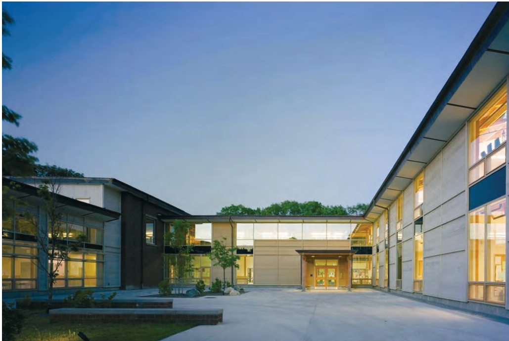
Wood End Elementary School, Reading, MA.
