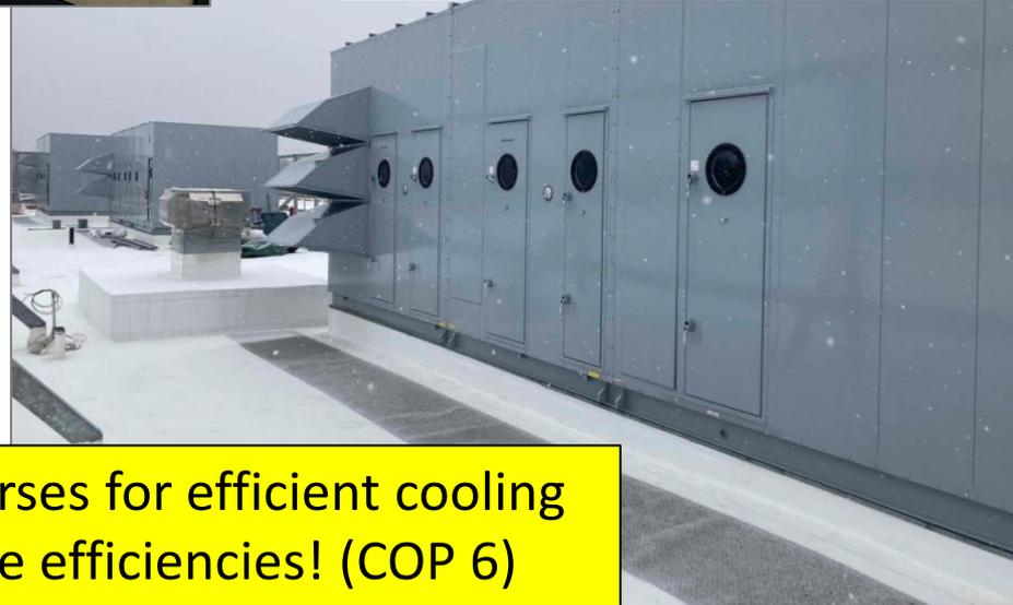
**Warm weather:** system reverses for efficient cooling
