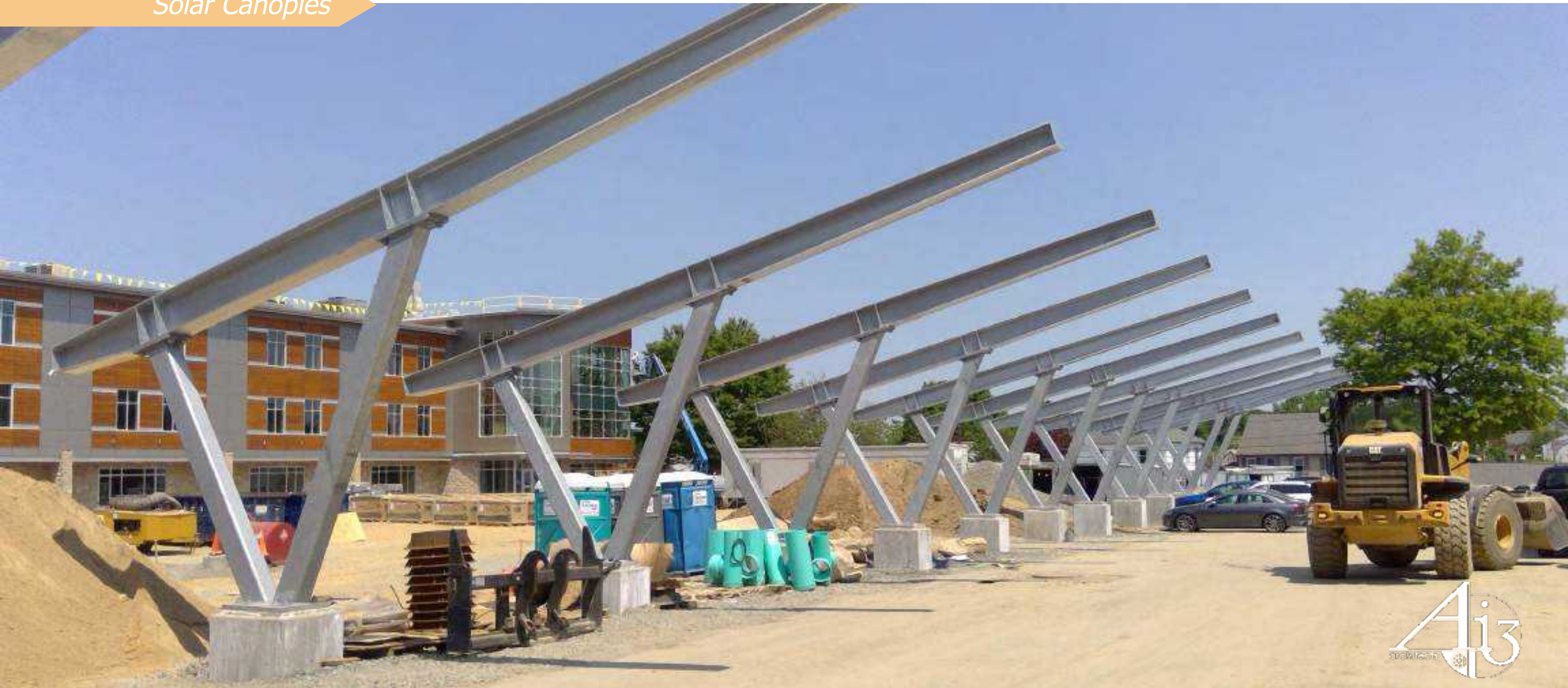
Installation of Cunniff solar canopy frames
